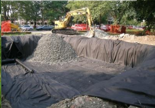
Sub-surface Detention Pond
